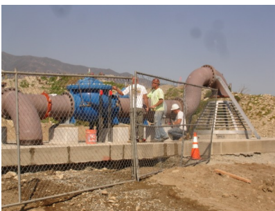
Installation of CB-14 Turnout
