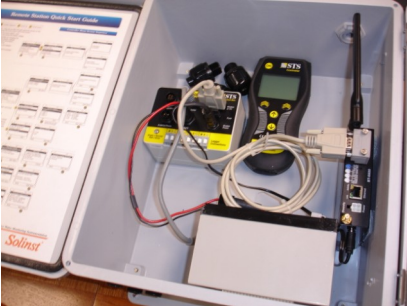
New Telemetry system being tested
